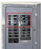
Circuit Breakers are a mechanical Over Current Protection Device [OCPD]. The OCPD is to protect the branch circuit feeds [wiring] and the appliances connected to them. Oversized breakers can damage the wiring and appliances. A qualified Licensed Electrician can help determine the safety of the Circuit Breaker box installation.
