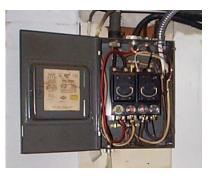
Fuses are an Over Current Protection Device [OCPD]. The OCPD is to protect the branch circuit feeds [wiring] and the appliances connected to them. Oversized fuses can damage the wiring and appliances. A qualified Licensed Electrician can help determine the safety of the fuse box installation.
